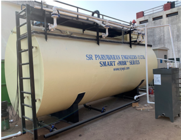
Carbon Steel Tank
